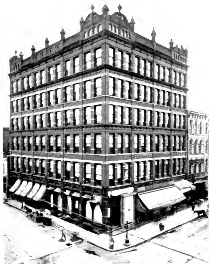
E. C. LAMB BUILDING
